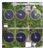
FIGURE 8-6 Aerial view of a water treatment plant that removes phosphorus from wastewater
